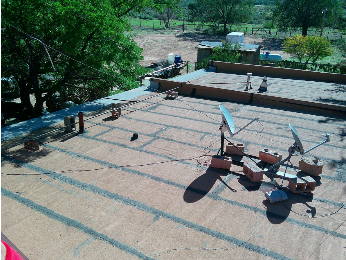
Figure 5. Rear roof section showing satellite dishes and roof penetrations
