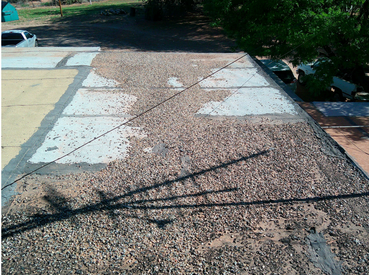
Figure 2. Gravel-covered roof section adjacent to the main roof.
