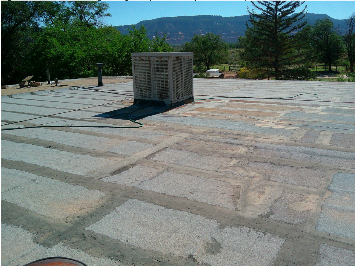
Figure 1. Roof surface showing existing swamp cooler, utility conduits, and penetrations.
