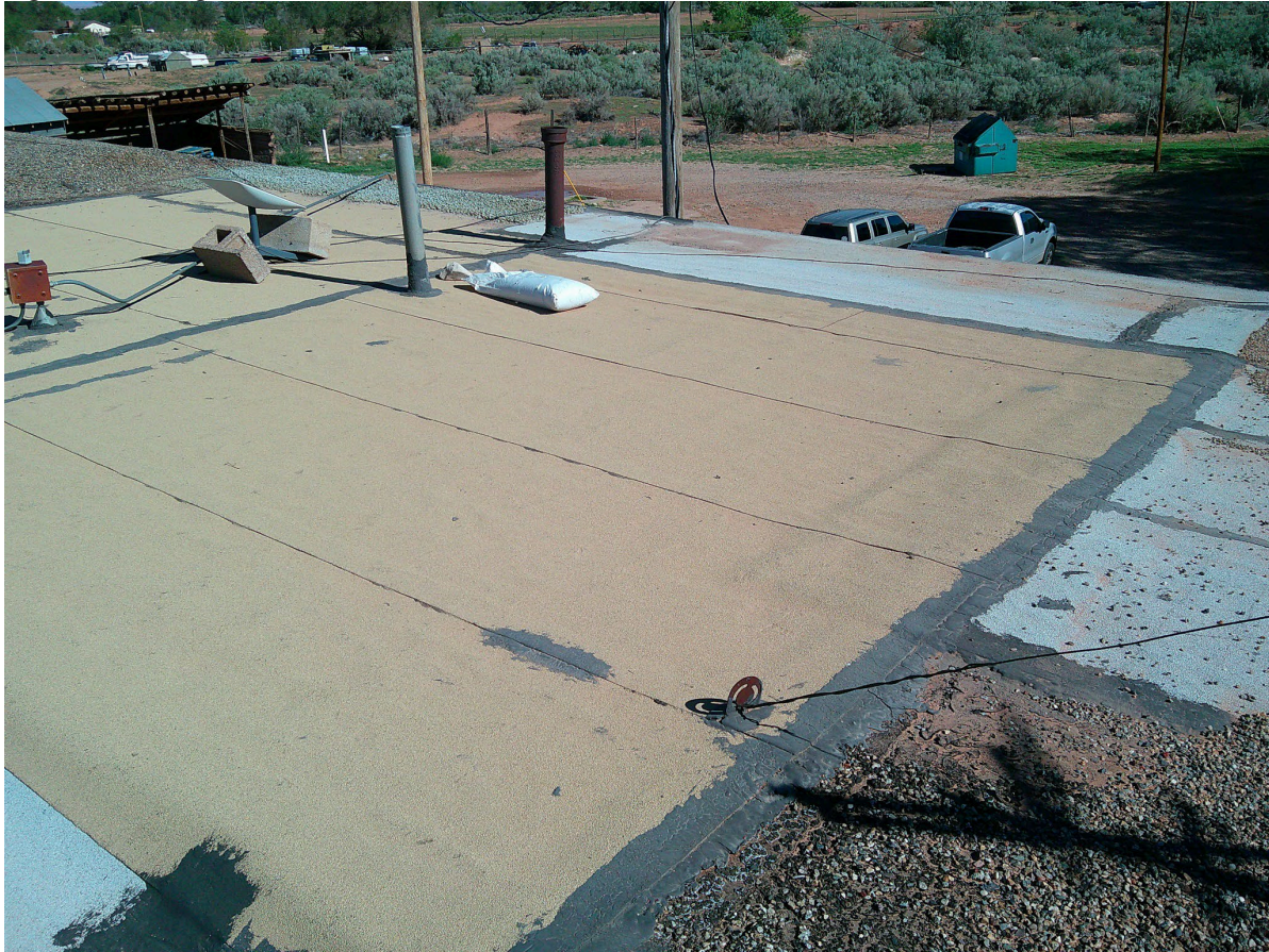
Figure 3. Existing roof membrane and transition between roof sections.
