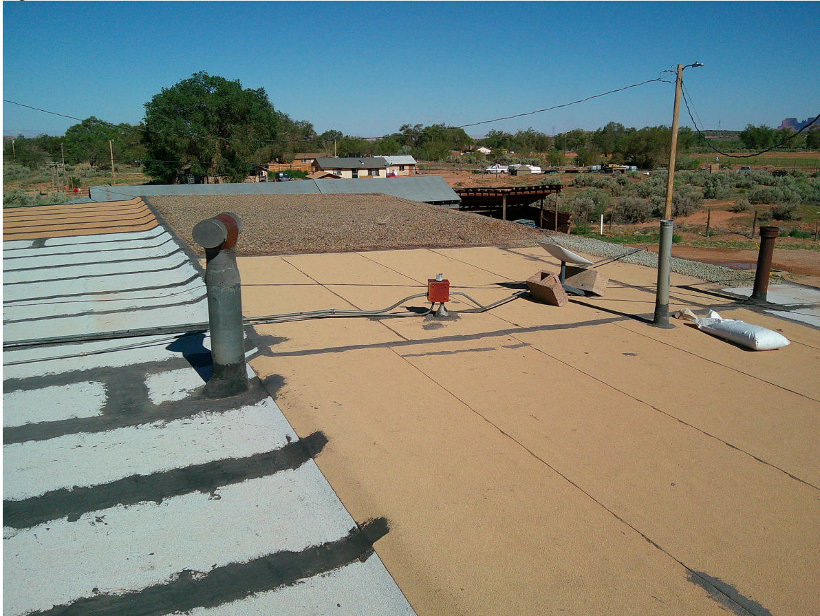
Figure 4. Overall roof condition from the northwest corner.
