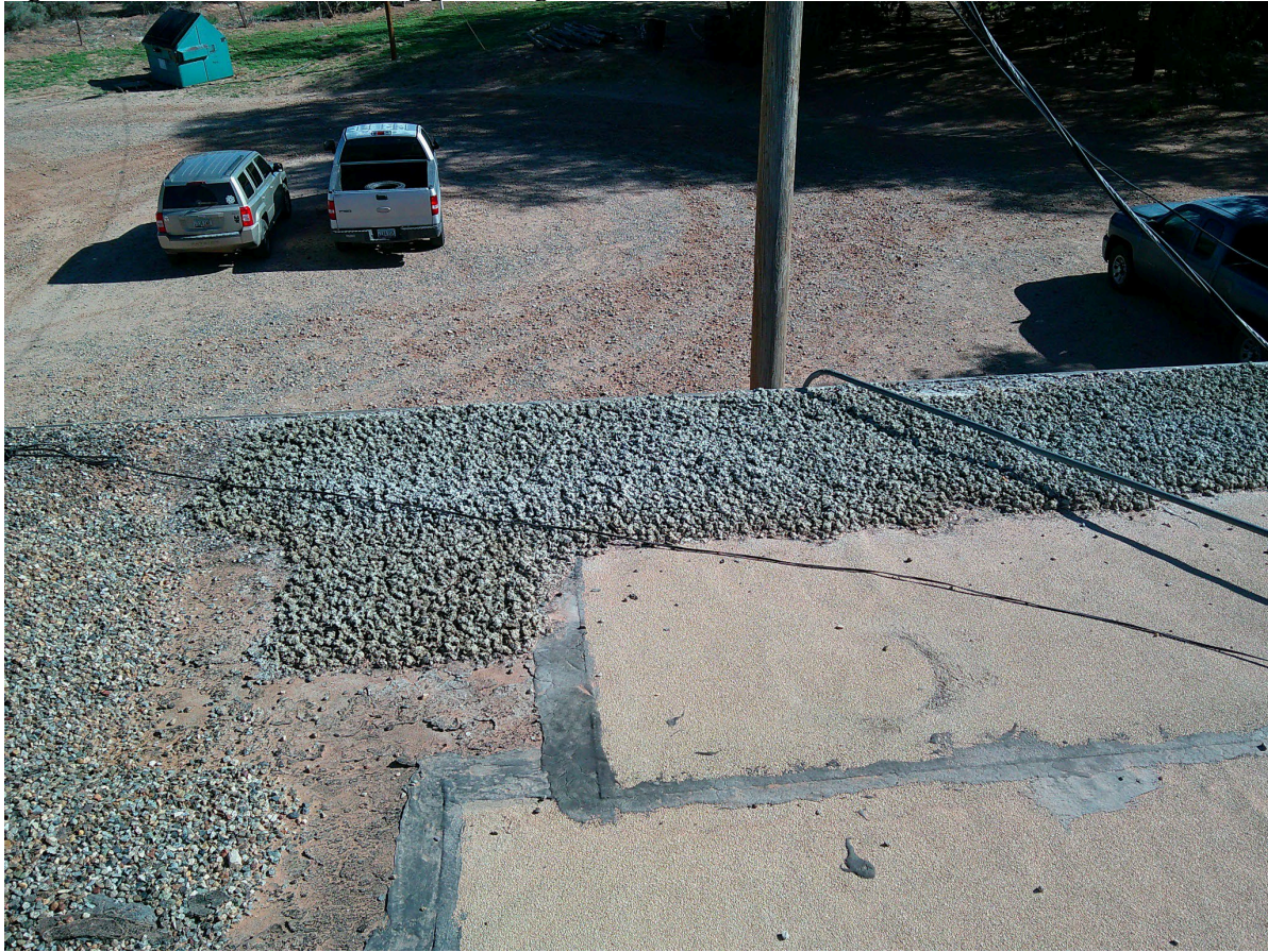
Figure 6. Rear roof section - existing gravel edge
