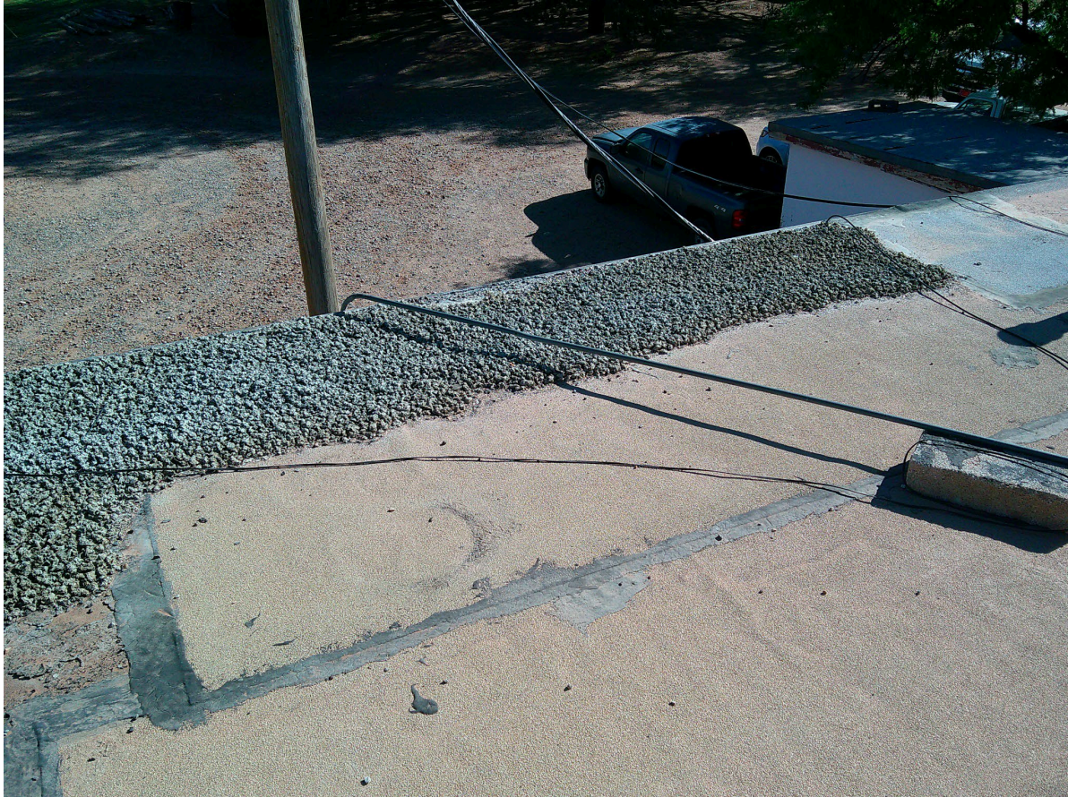
Figure 7. Existing gravel edge and roof termination detail.
